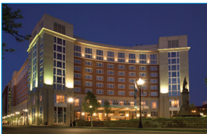
High Concrete Group produced energy-efficient, lightweight, durable, and aesthetically pleasing CarbonCast® facades for the award-winning Heldrich complex in New Brunswick, N.J.
