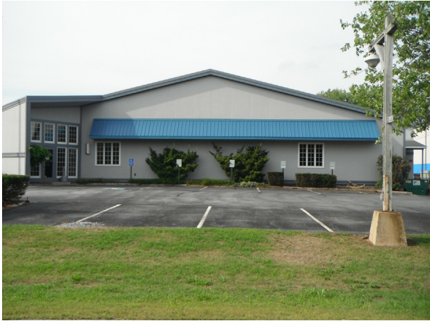
Building front facing Willow Street
