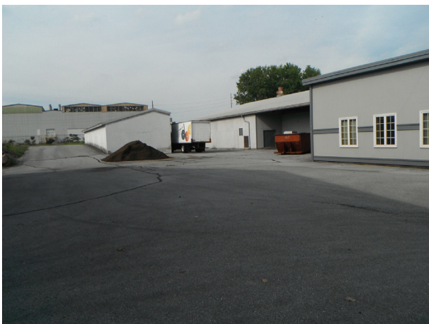
Outside storage on west side of warehouse/production area
