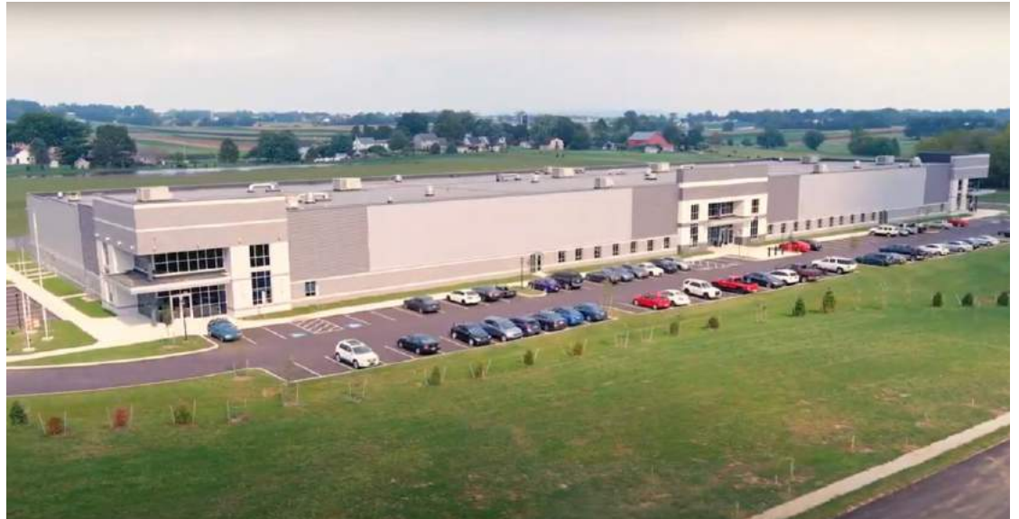
The new Thaddeus Stevens College Transportation Center in Greenfield was designed by Greenfield Architects Ltd. and built by High Construction Company.
